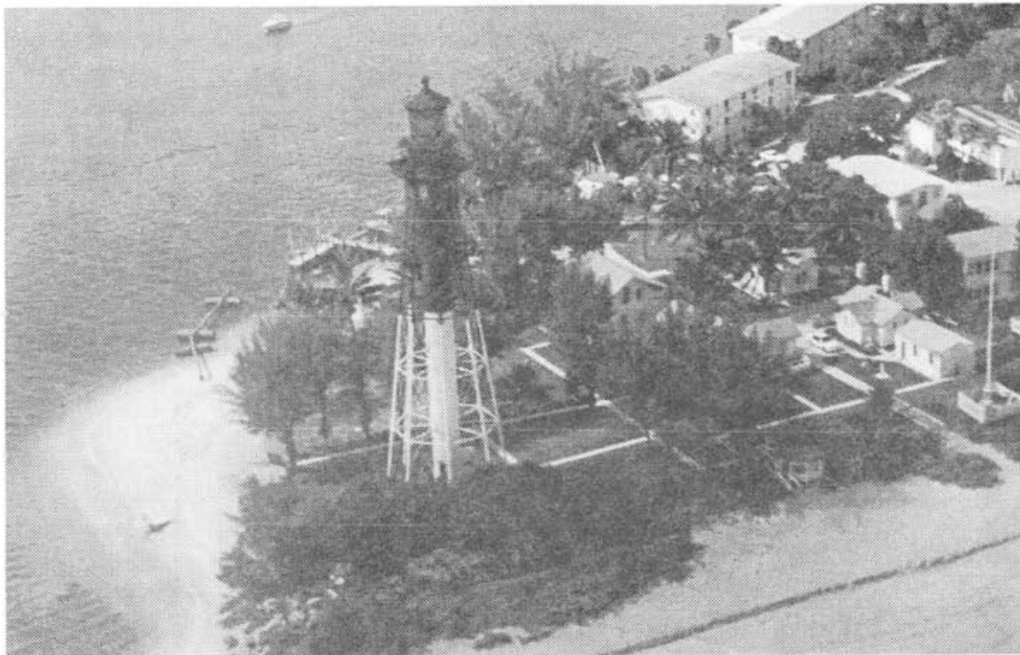
Early 1970's - Note the Radio Beacon Tower at far right, next to the Radio Room.
