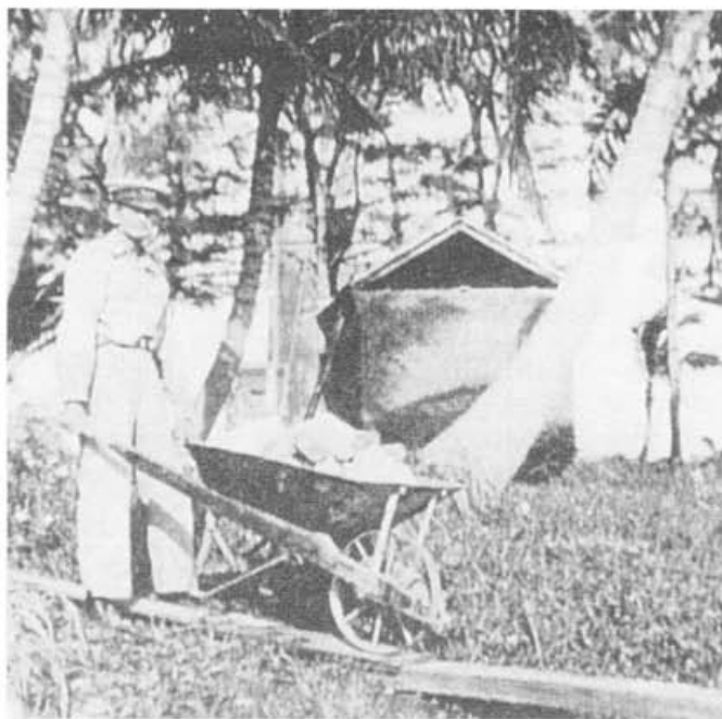
J. B. Isler dismantling the old brick oil house in 1938 after electricity came to the Station.
