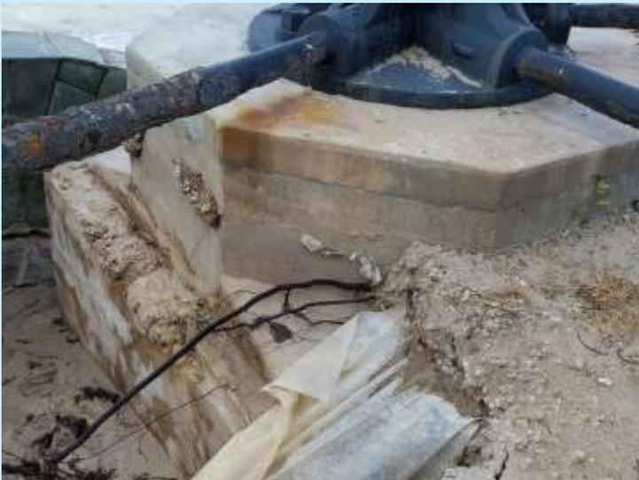
Photo #4—Footing Radial cracks
