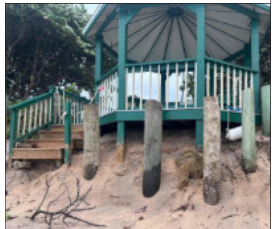
GAZEBO RETAINING PILINGS CIRCA OCT 2024
