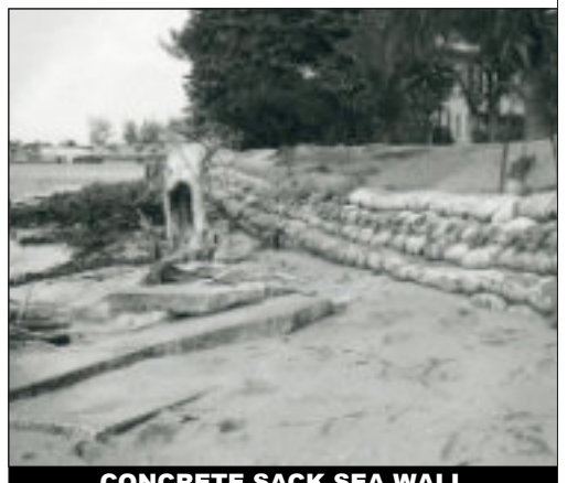
CONCRETE SACK SEA WALL CIRCA 1960'S
