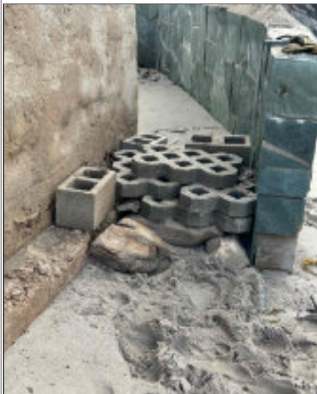
RETAINING WALL IN PLACE CIRCA OCT 2024
