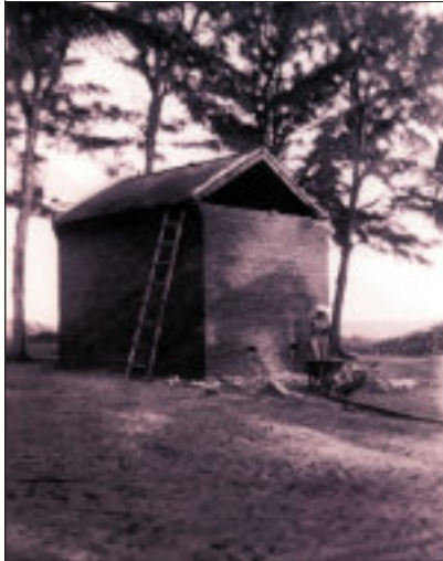
Dismantling of the oil house by JB Isler CIRCA 1930'S
