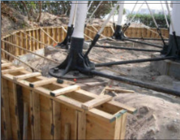
BUILDING THE RETAINING WALL CIRCA 2004
