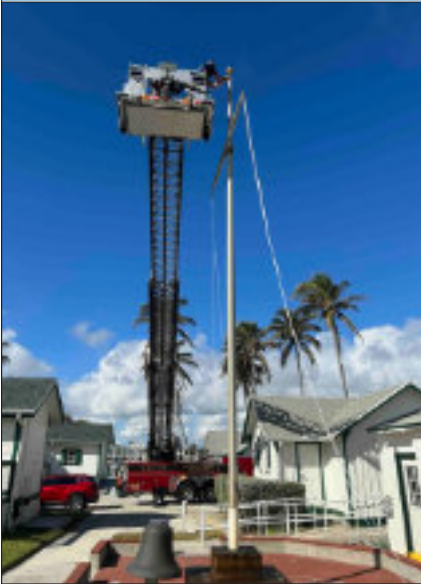
DEERFIELD BEACH FIRE RESCUE RESTRINGING FLAGPOLE CIRCA OCT 2024
