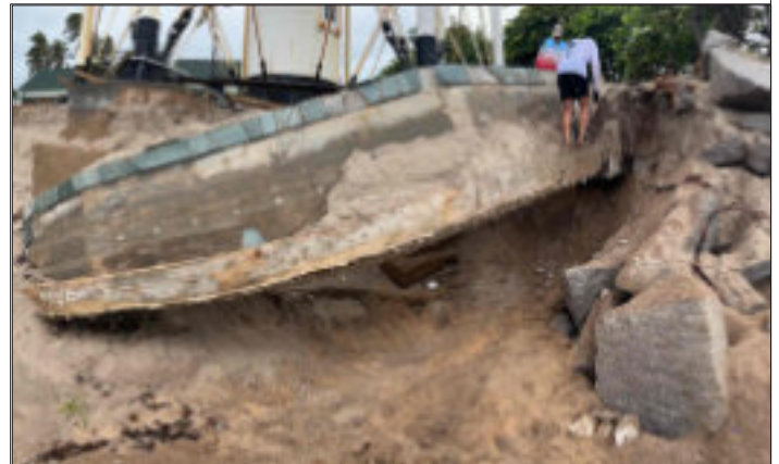
DROPPING THE RETAINING WALL CIRCA OCT 2024
